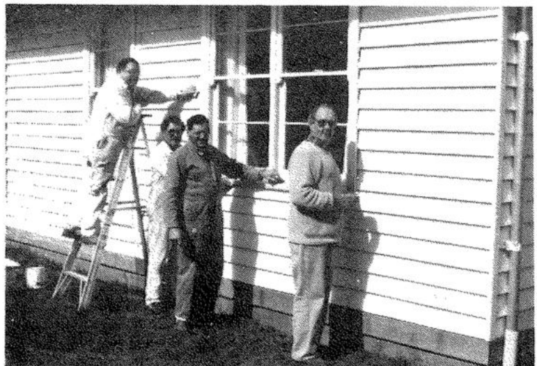
Volunteer painters (L to R): David Stone, John Murphy, John Ryan, and Bill Martin at work on the Cottage.
