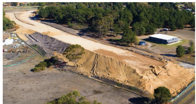
The earth formation for the bridge we're building over the Bellarine Railway.
